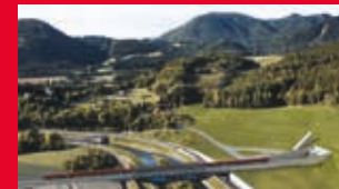
06 SEMMERING BASE TUNNEL 2012 - 2030
