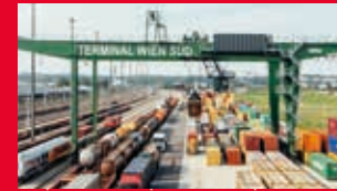
04 FREIGHT CENTRE VIENNA SOUTH 2013 - 2016
