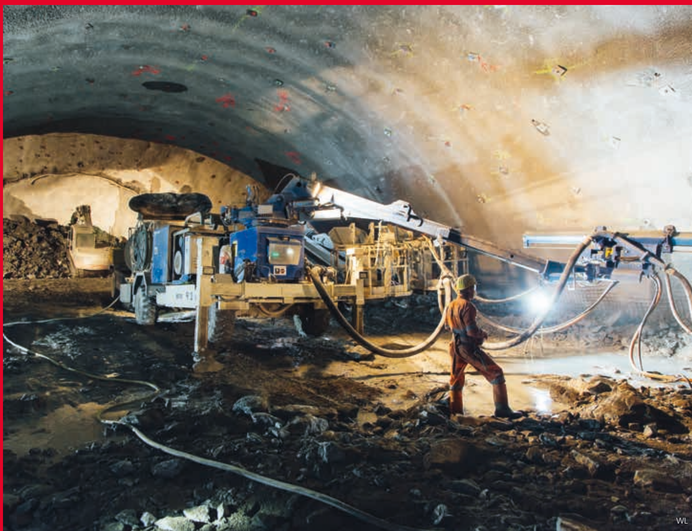
CONNECTING TUNNEL BETWEEN THE TWO MAIN TUNNELS, SEMMERING BASE TUNNEL
